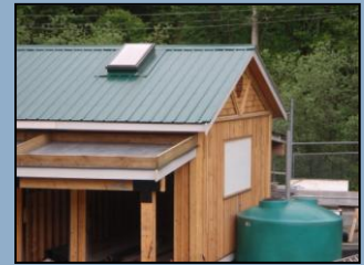
Allco green building, June 2010
