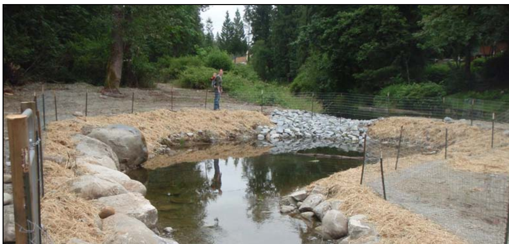
Above: 232 Street Channel retrofitted outtake with rip rap to ensure flooding will not occur and fencing to keep the beaver at bay.
