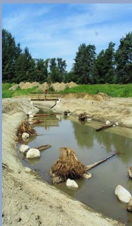
Trethewey Channel near completion
