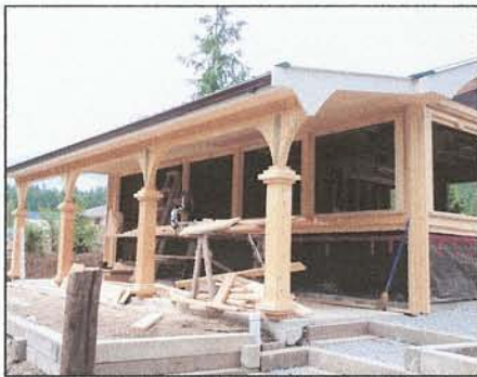
Construction of the new Allco Fish Hatchery office.
